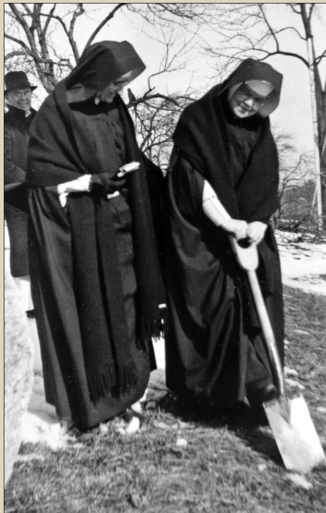
From the Centennial Archives: 1937—Mother Mary Gerald Barry and Sister Benedicta Marie Ledwidge break ground for the construction of new dormitory and dining facilities on campus, Archangelus and Benincasa Halls.
