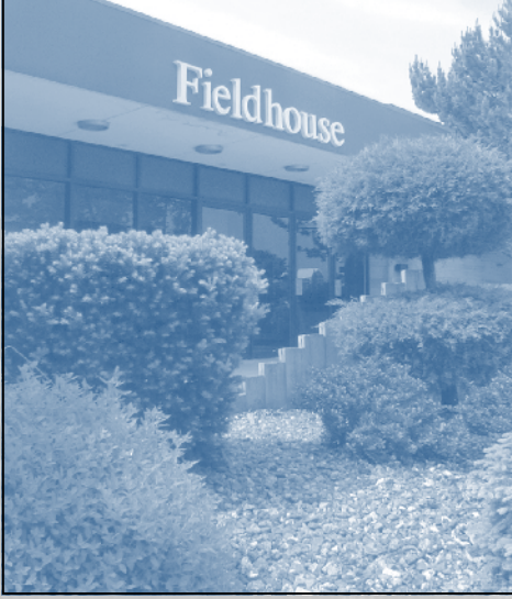
After 25 years the facade of the Fieldhouse is getting an update which will feature a new lobby.
