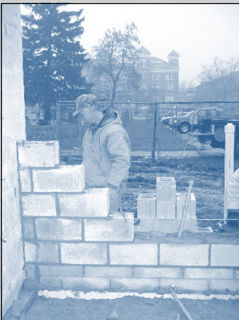
Jack Dominique builds a new fieldhouse wall. Photo date: 12/09/03.
