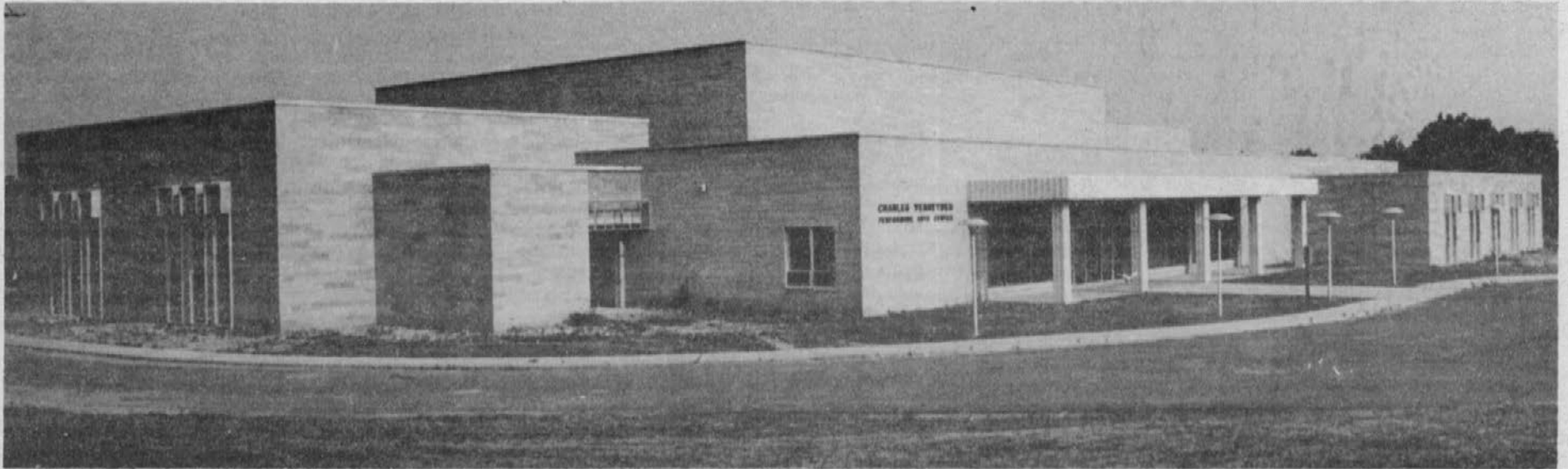
The Charles Verheyden Performing Arts Center just prior to the final touches of completion. The entire project took one year from the time of ground-breaking in October 1973 to dedication October 1974.
